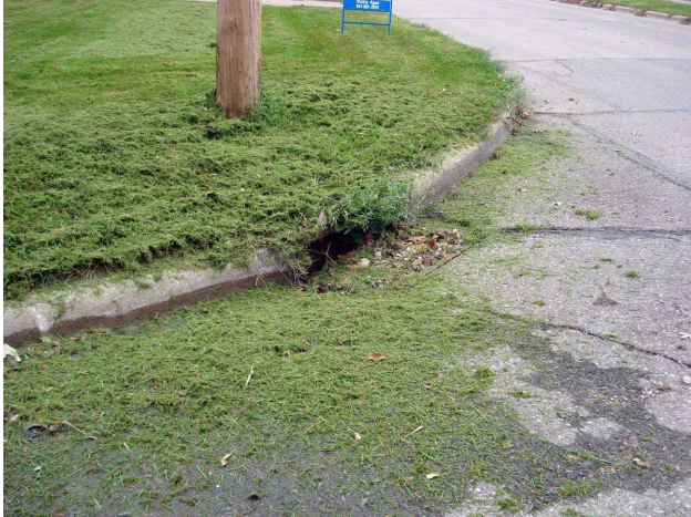
Figure 17. Grass clippings enter storm drains and carry excess nutrients to surface water.
