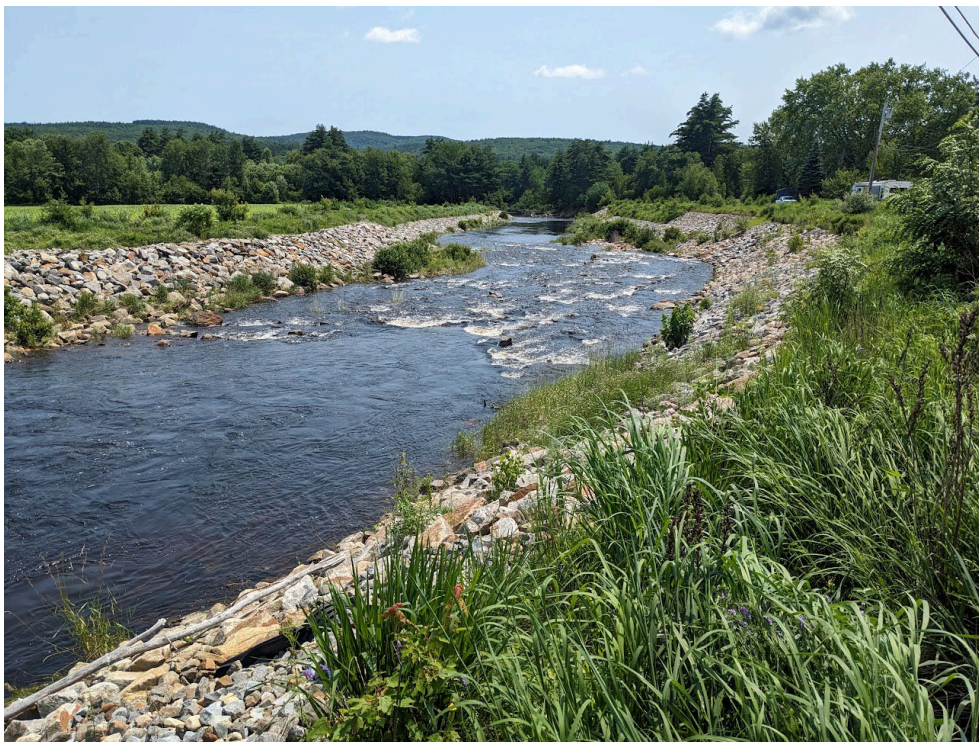
Figure 12. The Suncook River after extensive restoration efforts to stabilize the stream channel due to an avulsion during the 2006 Mother's Day flood.
