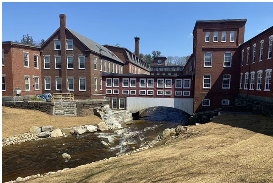
Figure 14. Sawyer Mill Dam post dam removal.
