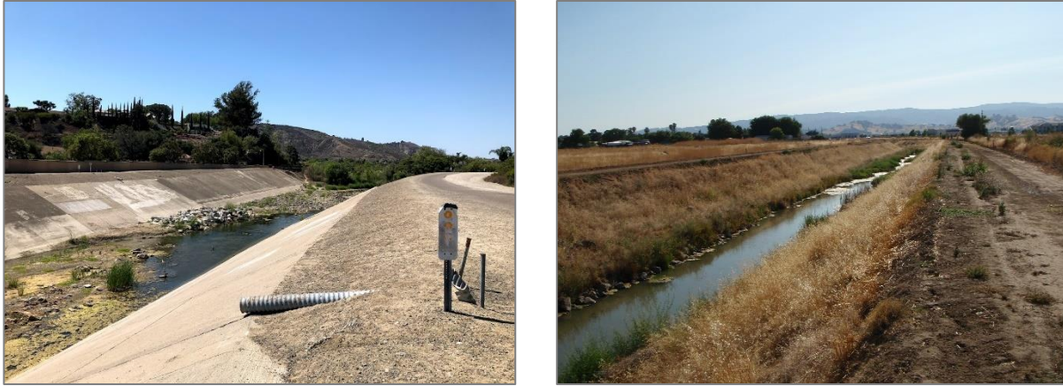
Figure 6. Examples of difficult conditions that may interfere with the observation or interpretation of indicators. Left: As the Arroyo Trabuco progresses through the city of San Juan Capistrano in California, its banks have been hardened and the natural riparian vegetation has been removed (although there is still aquatic vegetation apparent in the channel itself). The removal of in-stream and riparian zone habitat and addition of urban non-point source discharges may also impact the abundance of aquatic macroinvertebrates and hardened banks may obscure identification of bankfull elevation. Right: An unnamed creek near Vacaville, California, has been straightened and channelized, affecting naturally occurring stream pattern (e.g., riffle-pool sequence). Image credits: Raphael Mazor (left) and the California Department of Fish and Wildlife's Aquatic Bioassessment Lab (right).
