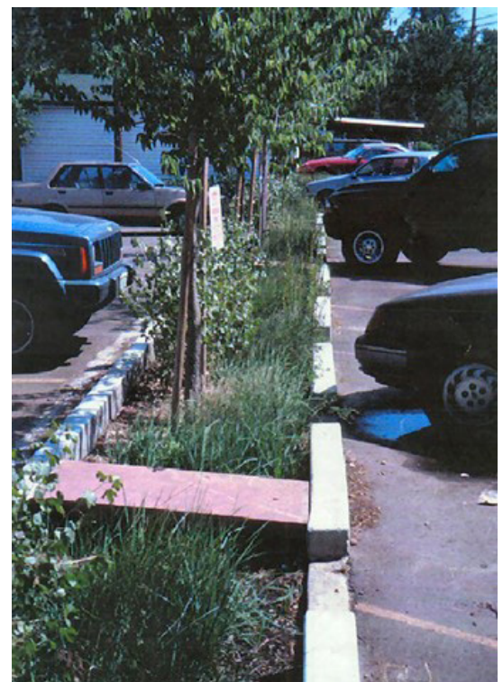
Raingarden solution to parking lot runoff.
