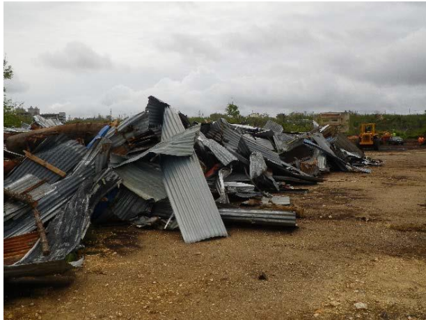
Figure 27. Corrugated metal roofing separated for recycling in a designated staging area after Typhoon Soudelor in Saipan.
