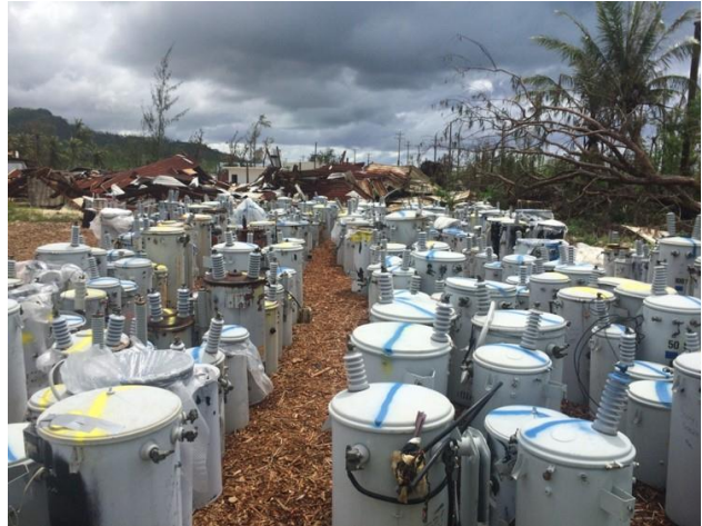
Figure 26. Waste caused by Typhoon Soudelor included 733 transformer carcasses and six drums of transformer oil contaminated with polychlorinated biphenyls, or PCBs.
