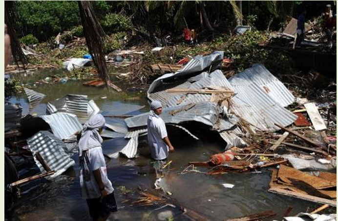
Figure 4. Two residents of the village of Leone, American Samoa, walk through waist-high water while removing structure debris after a tsunami (Casey Deshong / FEMA).
