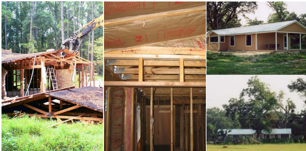
Figure 23. Panelized deconstruction was used to deconstruct a home in a floodplain buyout in Alachua County, Florida, and the lumber was used to build new Section 8 affordable housing inland (Brad Guy).
