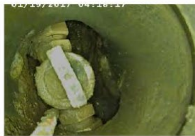
Non-Lead Service Line
