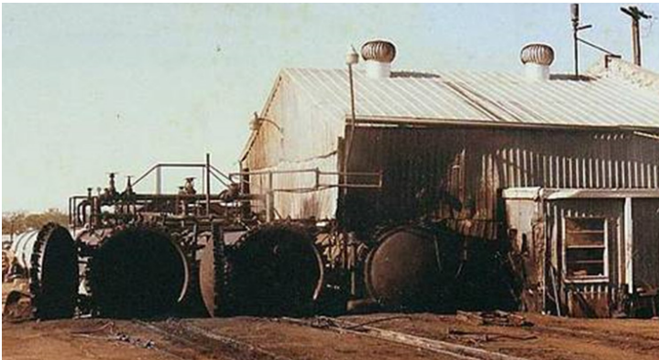
The former wood-treating facility on the Site.
