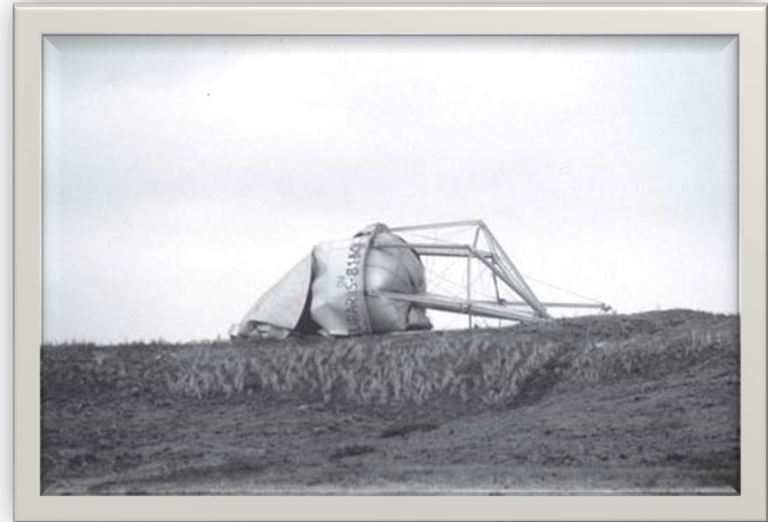
A water tower that has exceeded its useful life.
