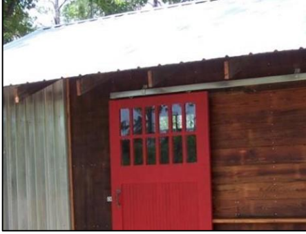
Nonprofit organizations built disaster recovery sheds after Hurricane Katrina to store recovery workers' belongings. The sheds were built entirely from reclaimed materials with the exception of the metal roofing. (Photos: Brad Guy)
