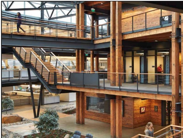
(Left): The Federal Center South U.S. Army Corps Seattle District Headquarters Building is a LEED Gold building completed by the U.S. General Services Administration in 2012 using 300,000 board feet of structural and nonstructural lumber from an adjacent warehouse that was deconstructed. https://www.gsa.gov/cdnstatic/GSA_FCS_Press_Book_email.pdf
