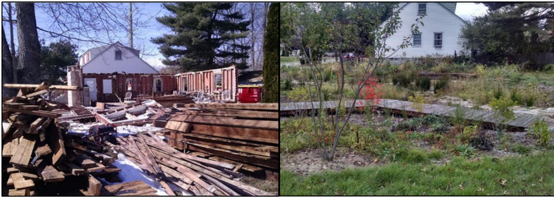
A home flooded during Hurricane Irene in New Jersey was deconstructed by Rutgers University Students and recycled concrete base and wood were used on-site to build a resilient floodplain pocket park. (Photos: Tobiah Horton)
