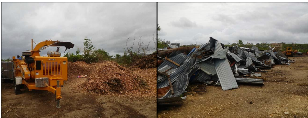
Clean green waste was mulched and given to residents and corrugated metal roofing was separated for recycling after Typhoon Soudelor in Saipan.
