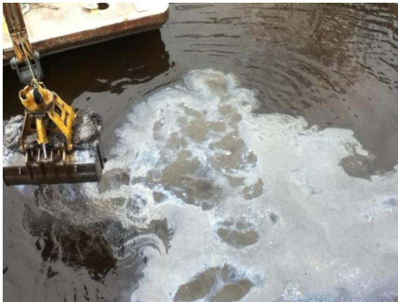
Picture 4. Dredging contaminated sediment at Camp Marina. (Photo taken by Stacy Hron, WDNR)
