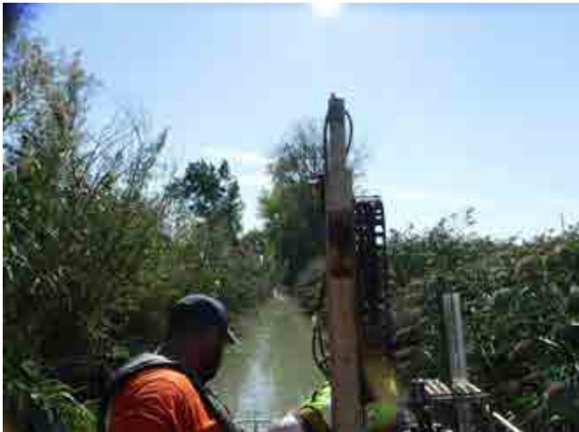
SD42 looking south.
