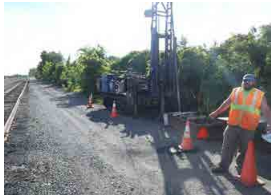
SO-07, Rig Placement (14' bgs).
