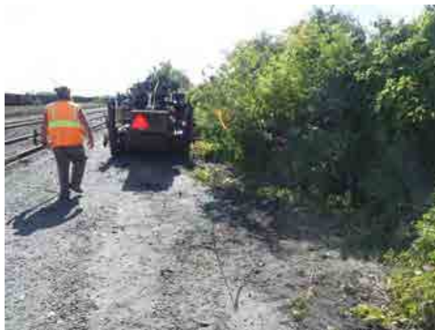
SO-08, After Drilling Activities.
