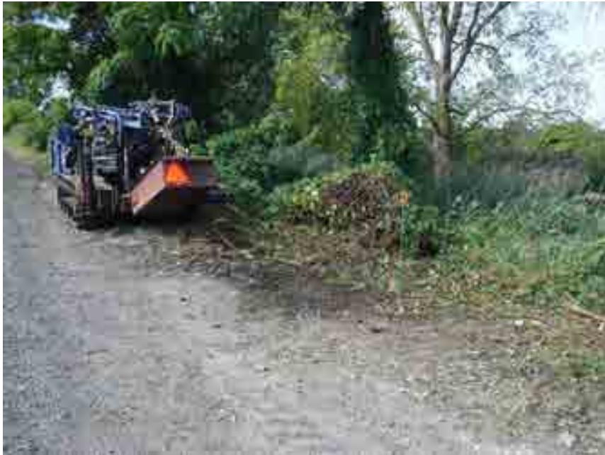
SO-09, After Drilling Activities.
