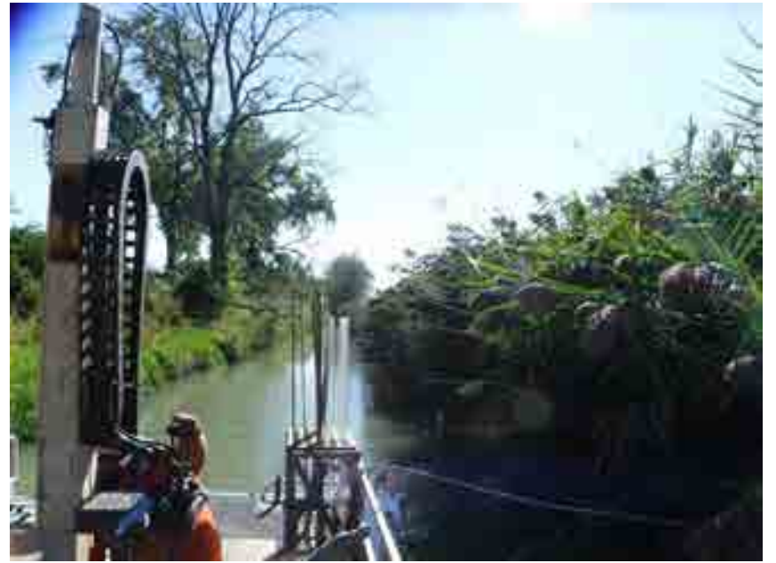
SD41 looking south.
