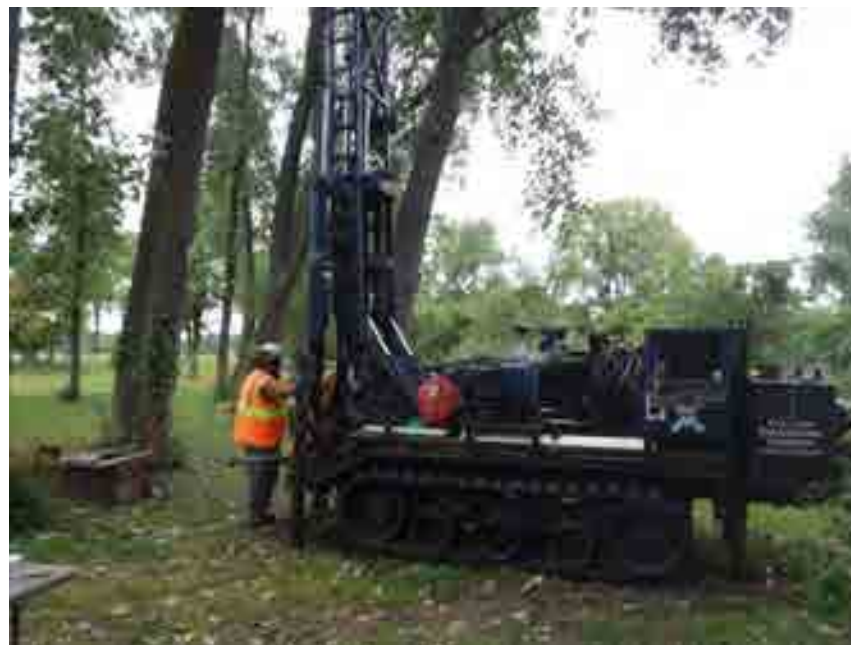
SO-01, Drilling Activities.
