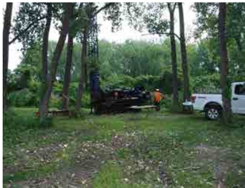
SO-01, Removing Augers.
