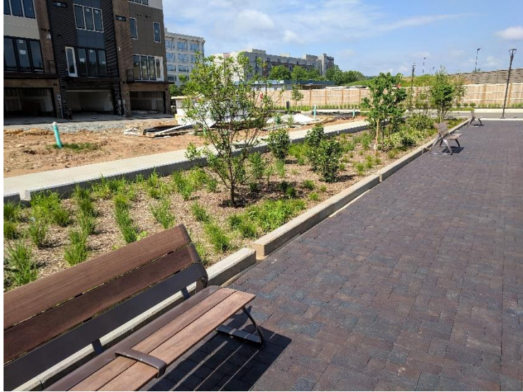
Figure 30. SCM integration into the landscape of a residential development site in Alexandria, VA.
