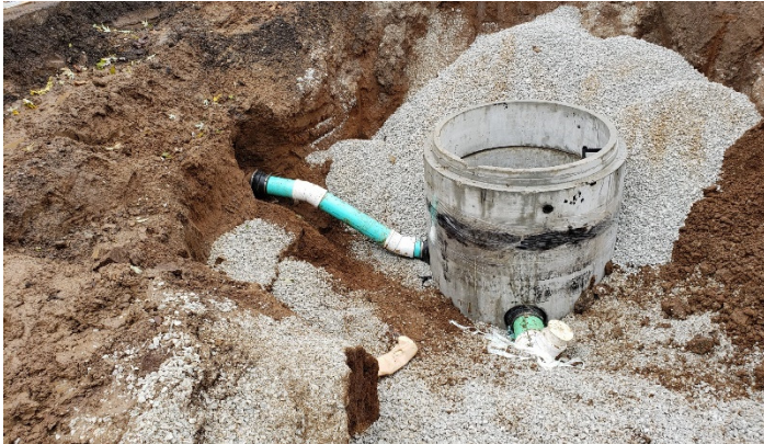
Photo #1: Looking southwest during installation of new sewer manhole structure #5 (MH #250053)
