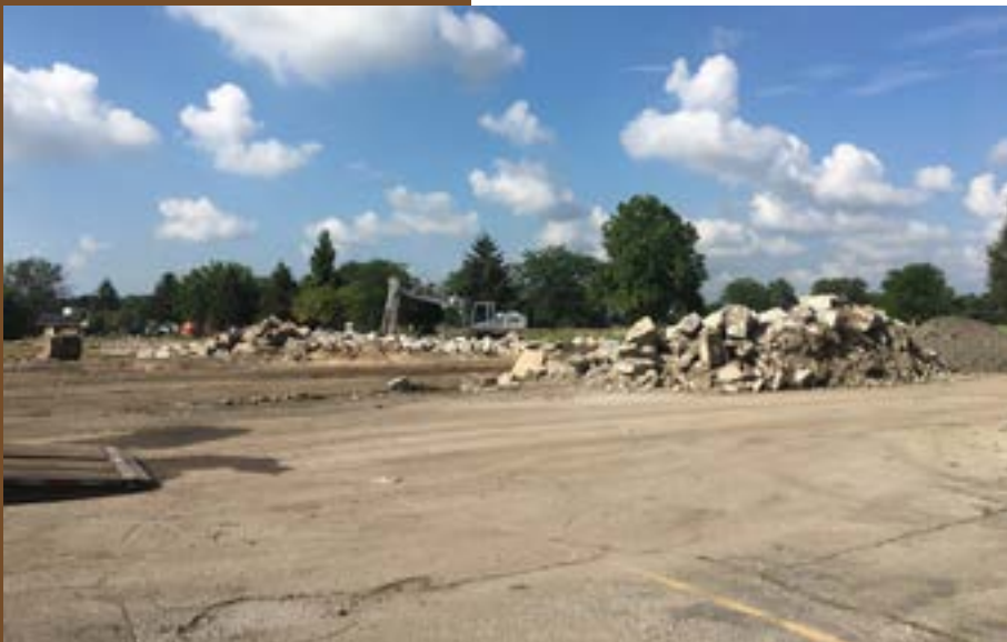
Demolition of Zone 1 nears completion.
