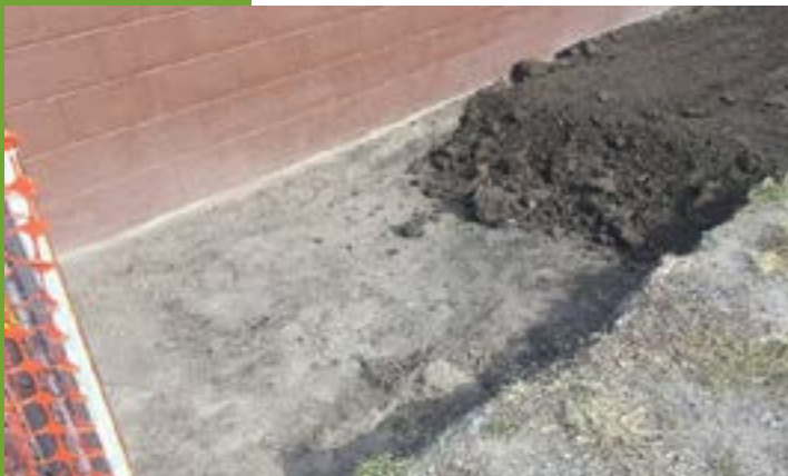
Clean soil is placed after excavation.
