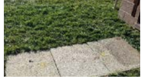
New sod is placed to restore yard.
