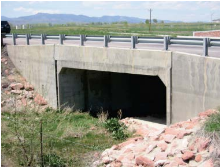
Figure 3-2 Concrete Box Culvert
