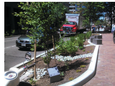
This bioretention cell was retrofitted into the right-of-way to capture stormwater from the street.
