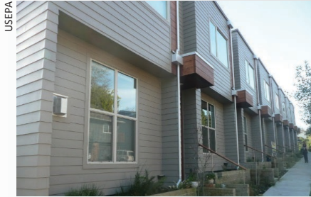
USEPA Roof runoff enters bioretention flow-through planters for treatment and short-term storage.
