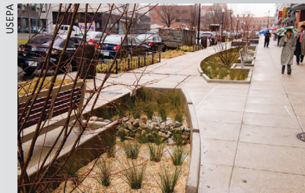
USEPA Runoff flows into stormwater planters installed in the sidewalk adjacent to benches.
