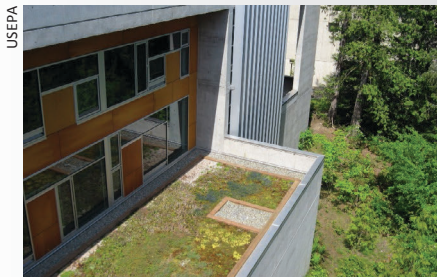
USEPA A building's green roof captures rainfall, thereby reducing local runoff.
