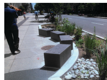
Benches provide public seating while also discouraging damaging foot traffic through the stormwater bioretention cell.
