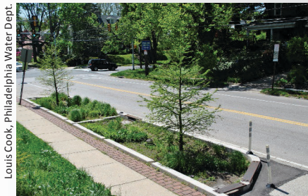
USEPA Louis Cook, Philadelphia Water Dept. This stormwater curb bump-out intercepts stormwater runoff flowing down the street.
