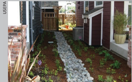
USEPA Roof downspouts direct runoff water to rock swales between homes.
