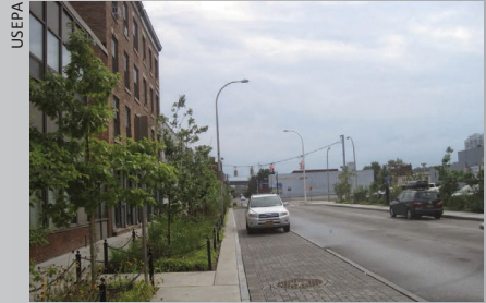
USEPA A permeable interlocking concrete paver parking lane is adjacent to a sidewalk planter.
