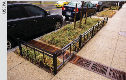
USEPA A bioretention cell receives stormwater runoff through a curb cut and surface grate.
