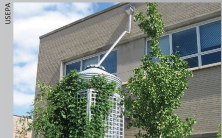
USEPA A cistern collects rooftop runoff, which is used to water landscape areas around the building.
