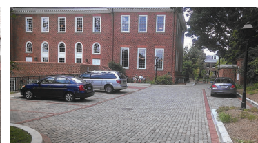
A permeable-paver parking lot allows stormwater to infiltrate while preserving parking spots.
