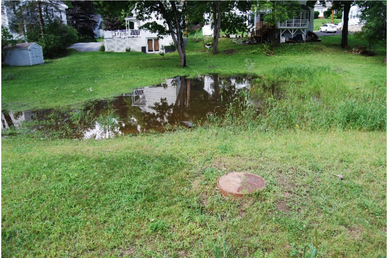
Figure 2-1. Low-lying areas experience frequent ponding of stormwater from upslope areas and occasional sanitary sewer overflows
