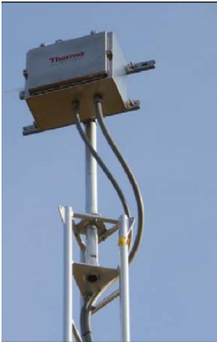
NO y Converter at 10 meters
