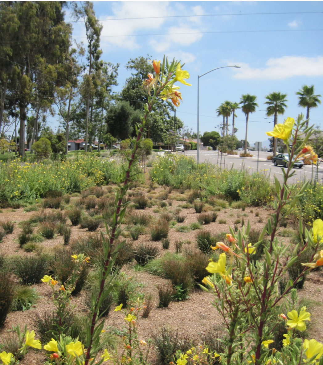
Photo courtesy of Jason Wright, Tetra Tech Bioretention in Albuquerque
