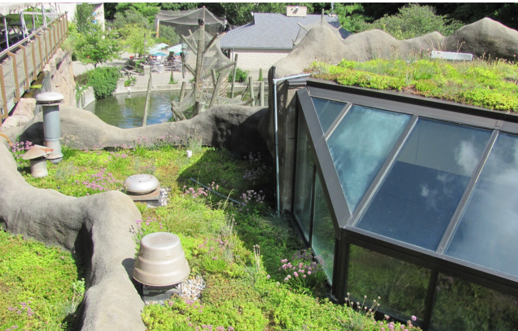
Photography courtesy of Dan Christian, Tetra Tech A green roof over an exhibit at the John Ball Zoo in Grand Rapids.
