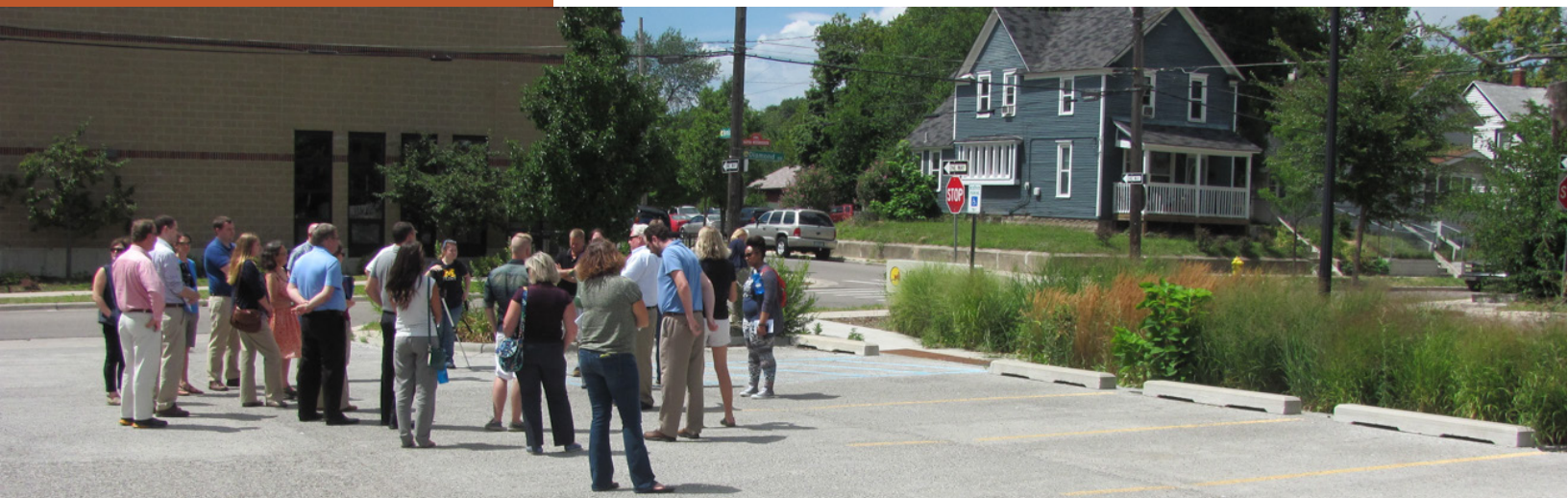
Photography courtesy of Dan Christian, Tetra Tech Porous concrete parking lot and bioretention at Joe Taylor Park in Grand Rapids.
