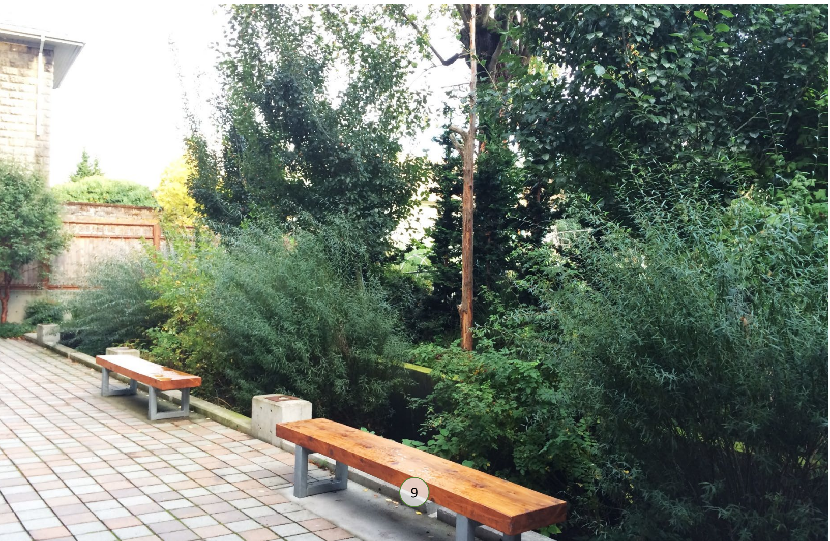
A courtyard bioswale serves dual purposes as stormwater management and attractive landscaping
