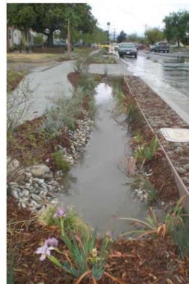
Stormwater flows through a curb inlet into a bioswale on Elmer Street. The water infiltrates into the soil within a day, preventing breeding mosquitoes.
