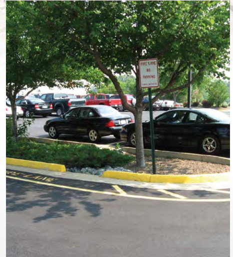
In this Virginia parking lot, traffic islands are designed with curb-cuts and a porous drainage medium to allow runoff to collect and infiltrate.
