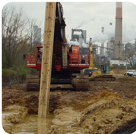
Excavation of a slurry wall trench
